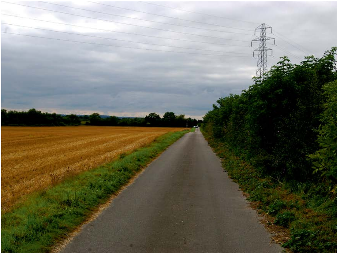
Fig 15 Boundary Road looking west (MOLA photo 12.09.2013)
